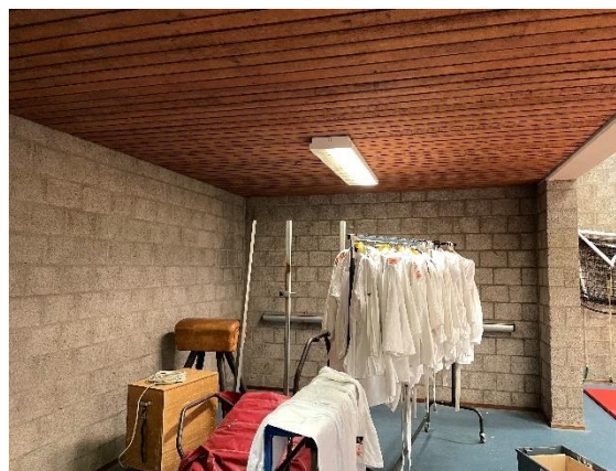
plafond berging, gymzaal 4
