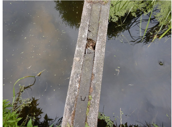
Figuur 4.27: Houtrot in plank object X1072
