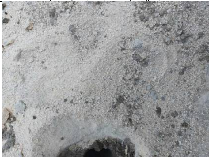
Foto 9: Zandcement traject 0,0 – 0,1 m-mv (boring 30)
