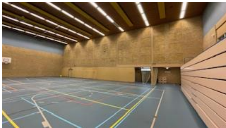
Foto 3: Interieur hal; links is achtergevel
