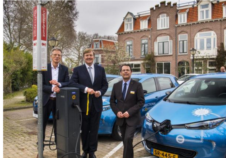
Smart Solar Charging
