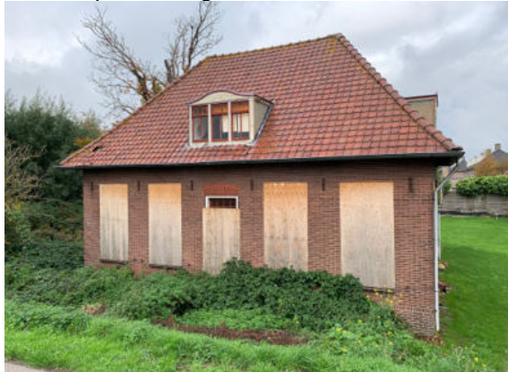
De te slopen woning.
