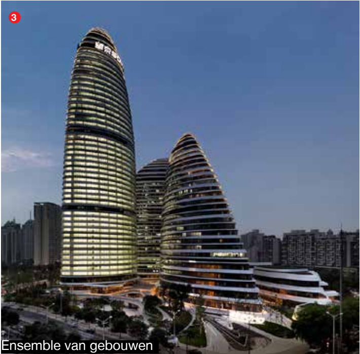
Wangjing SOHO, Beijing
