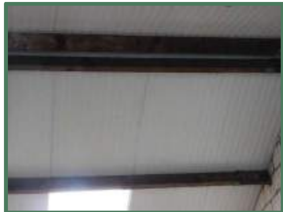
Sandwichpanelen dak te slopen loods
