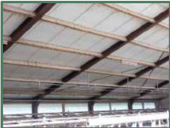
Sandwichpanelen dak rundveestal
