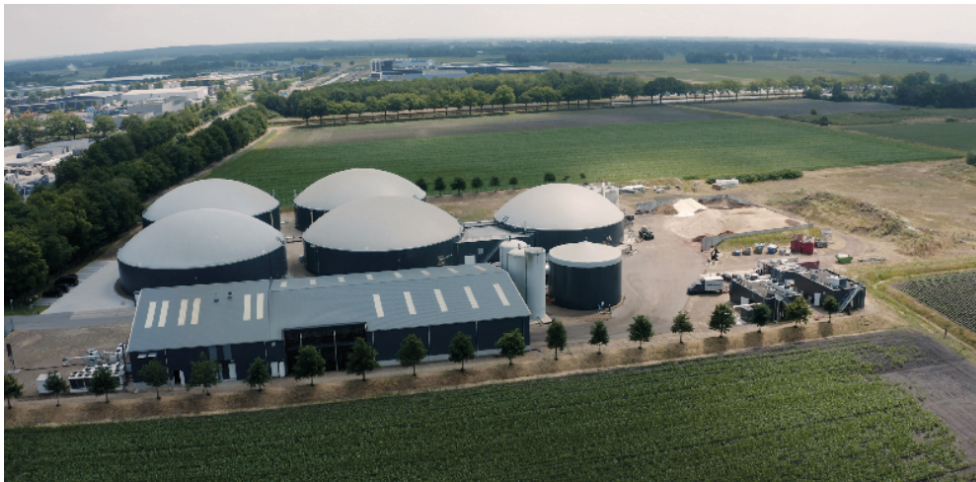
Figuur 4.18 Groen gasinstallatie in Hardenberg (bron: https://www.engie.nl/over-ons/kennisbank/nieuws/240416-overname-groen-gas-installaties )
