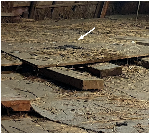
Figuur 8. Latrine steenmarter, 2 e verdieping.
