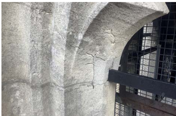
35.5 scheur in tracering open geleding middentoren
