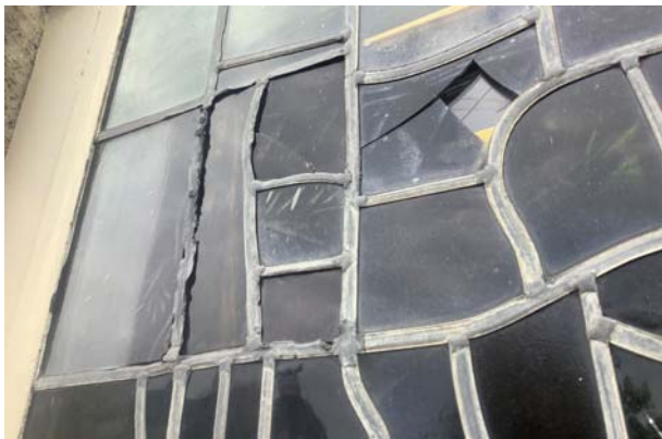
34.2 g-i-l panelen westgevel
