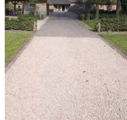
oprit in halfverharding
