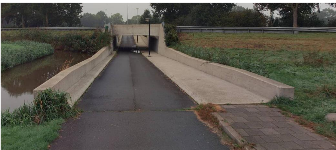
Figuur 23: Fietstunnel Hakkelbout, Nieuwkoop N231 ( https://streetsmart.cyclomedia.com )
