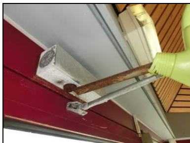
Corroderende deurdranger
