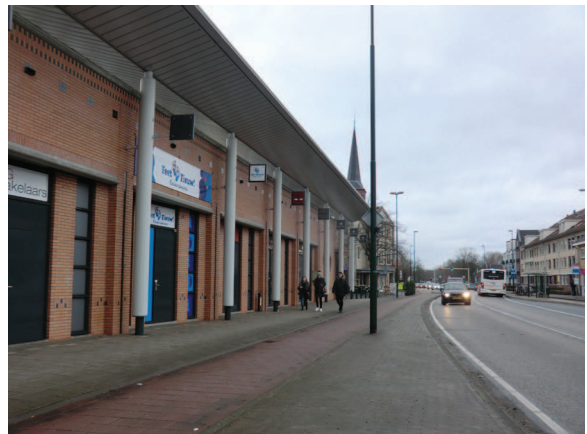
Fig 3.5.3.4 - "De muur" in the center of Aalst
