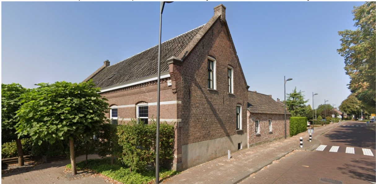
De oude school in 2020. GOOGLE STREETVIEW.
