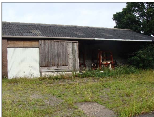
Foto 4. Te slopen loods
