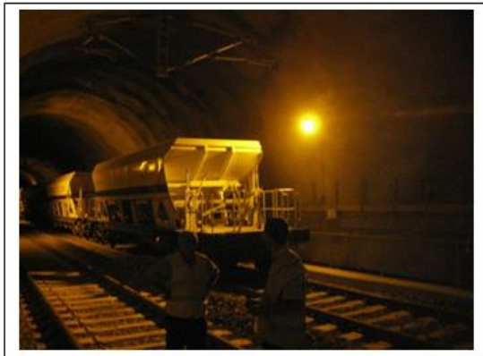
Inside the tunnel. The excavation and lining is fully complete as is the coating, waterproofing and drainage.
